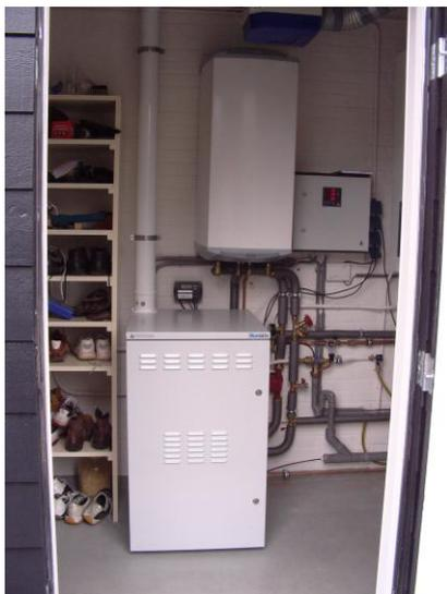
*Figure 4-3: The CFCL BlueGen installed in an installation room. De CFCL BlueGen stands on the floor and there is a 100 liter warm water storage on the wall.*
